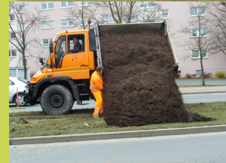
Fig. 2: Installation of the FLL-substrate for open tree pits
